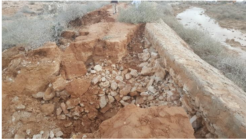
Figure 12. Sedimentation in front of one of the diversion barriers
