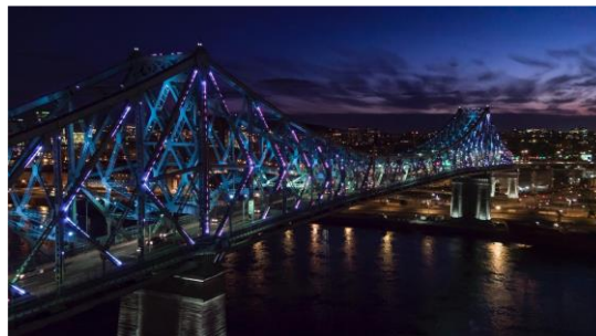
Figure 7. Living Connection Bridge (Source: Alexandra, 2019)
